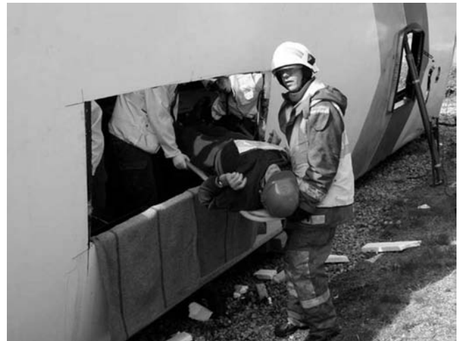
Figure 18.17. Cutting an opening in the roof, which is feasible in 2 minutes with a circular saw, facilitates evacuation. This intervention permits ambulance personnel to work in the passenger compartment and to evacuate victims by using the most appropriate exit pathways. See color plate.
