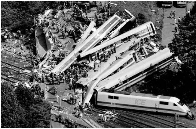
Figure 18.9. The Eschede, Germany, train disaster is one of the world's worst high-speed train disasters. The train disintegrated in the crash and the disaster claimed 101 lives and injured 103. See color plate.
