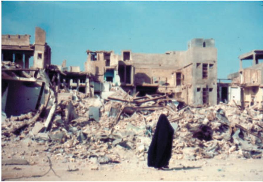
Plate 24.4.2. “Collateral damage” goes beyond injury and death. The fragile and superficially placed piping seen in the foreground was the main water artery to this village in Iraq. Public health infrastructure may be different than the normal standard for civilian contractors, the military, and aid workers. Public health “indirect” deaths are more prevalent than direct deaths from weaponry and violence. (Burkle, 1992)
