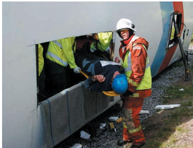
Plate 18.17. Cutting an opening in the roof, which is feasible in 2 minutes with a circular saw, facilitates evacuation. This intervention permits ambulance personnel to work in the passenger compartment and to evacuate victims by using the most appropriate exit pathways.
